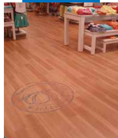
Solid Timber Flooring installed over Ultraplan Eco in a Pumpkin Patch store in Sydney, Australia
