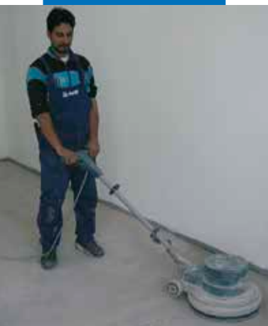
Polishing with helicopter before applying Ultraplan Eco - Mirabello kindergarten - Cantù (Como) - Italy
